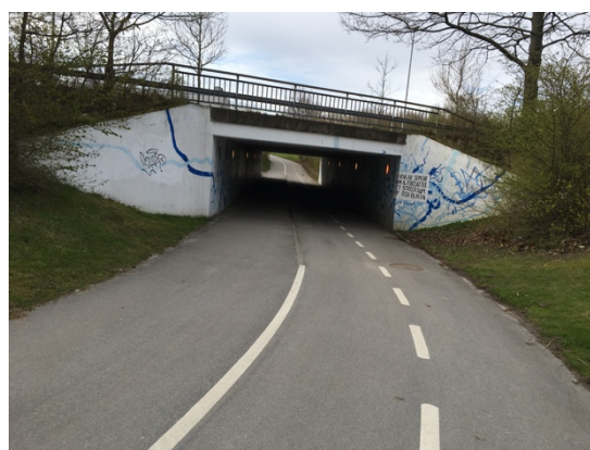
Figur 11. Tunnel under Getingevägen.
