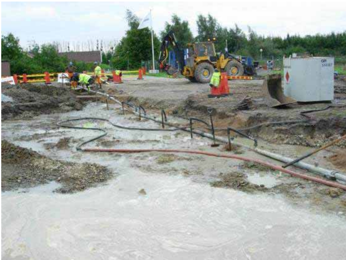
Figur 4.12 Västra Gryet – wellpoint
