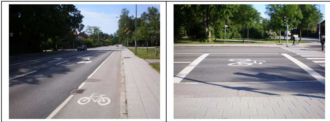
Figure 17: Site Type A at Tunavägen East, signalised intersection of Tornavägen-Tunavägen (left) and bicycle box for waiting bicycle during red light (right)
