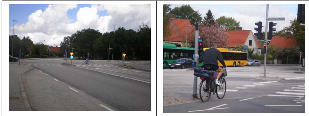
Figure 18: Site Type B at Tornavägen South, signalised intersection of Tornavägen-Getingevägen- Svenshögsvägen (left) and signal facility for cyclist when crossing (right)
