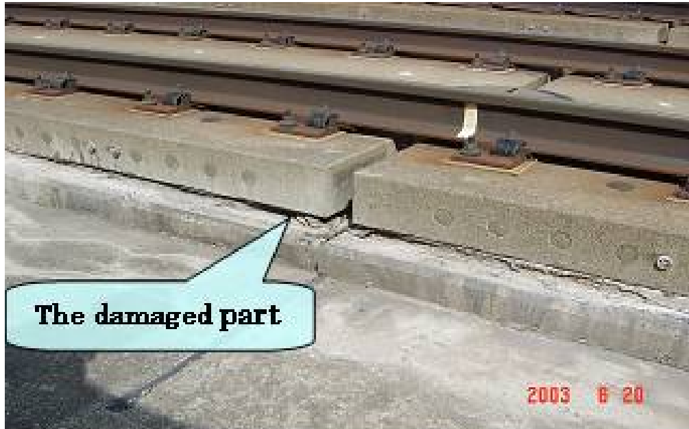
Figur 18, hur sprickbildning i cementasfaltsbruket under plattan (Yokoyama, 2007)
