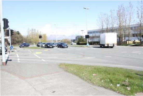
Figure 3-21 Intersection at Grensásvegur
