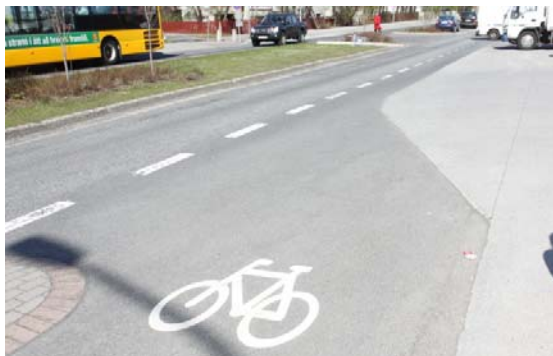
Figure 3-13 Indented cycle lane at intersection
