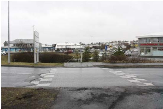
Figure 3-6 Elevated crossing in Skeifan
