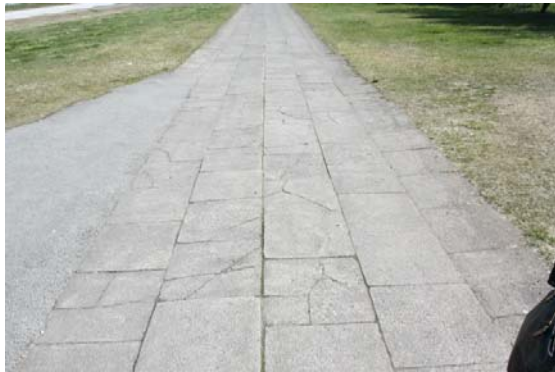
Figure 3-16 Uneven surface
