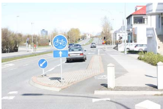
Figure 3-14 Cycle lane approaching intersection
