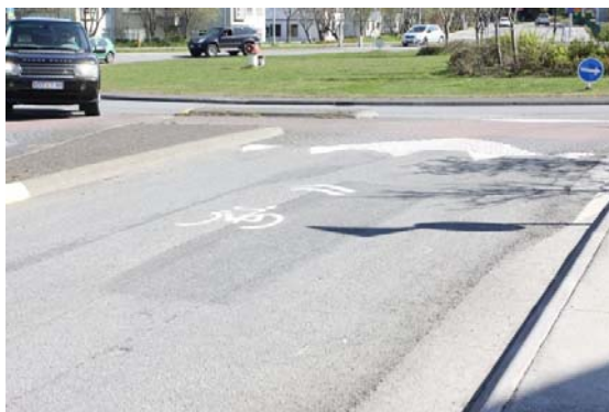
Figure 3-11 Cycle sharrow at the entrance of a roundabout
