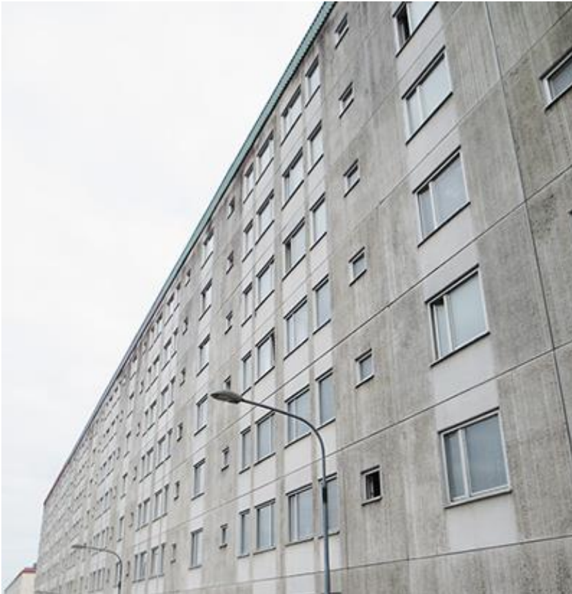
Figure 1.1. Typical façade of a dwelling from the 1970 th with an element built façade construction (Adapted from www.byggteknikforlaget.se ).
