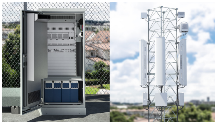
Figure 2.3: Ericsson 3-sector RBS with cabinet enclosure to the left containing baseband, batteries and climate control. Right side shows three antennas with 3 remote radio units.
