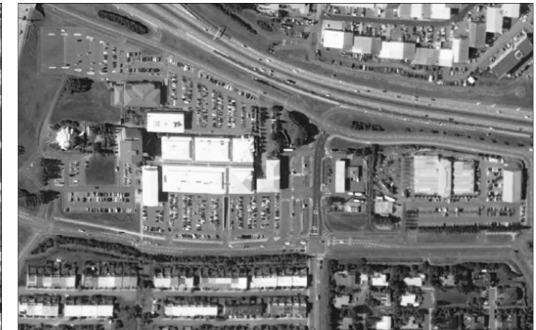
56. Mjóddin service center., the design site.
