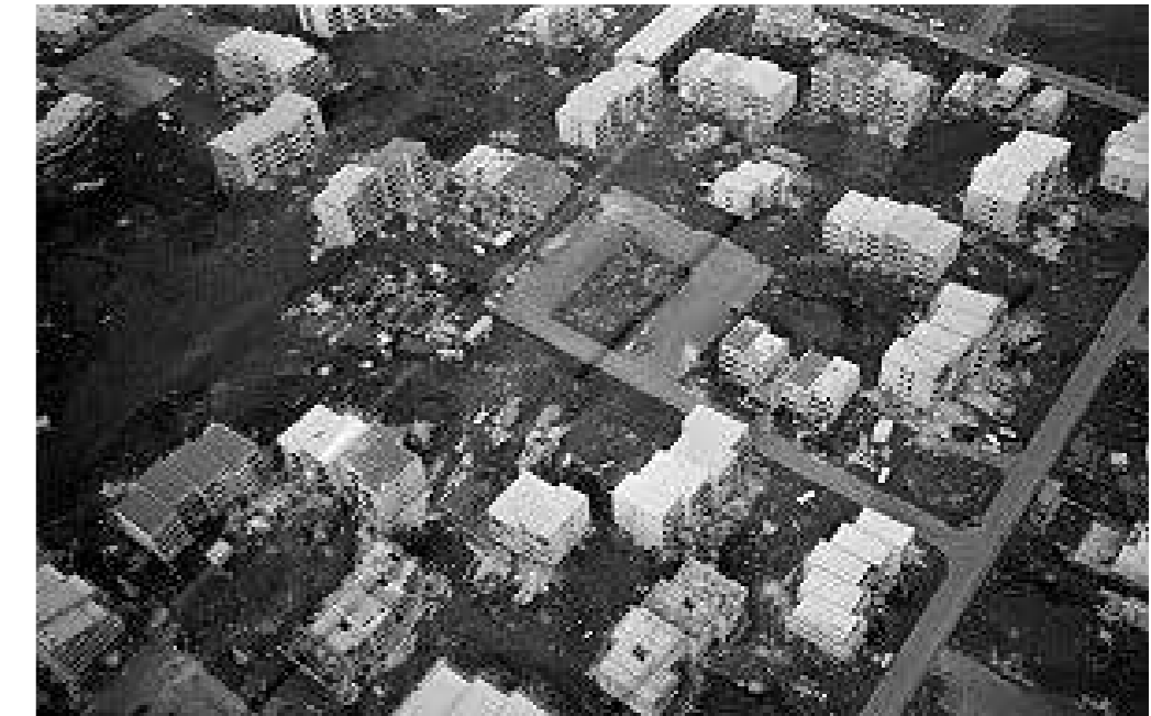
102. Seljahverfi under construction 1976.
