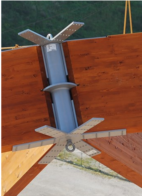
(a) Connection in one of the Brindisi domes, from R. Crocetti [65] .
