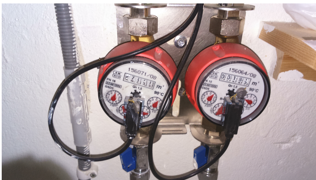
FIGURE 3.5: Installed water meters at the incoming pipe to the kitchen.
