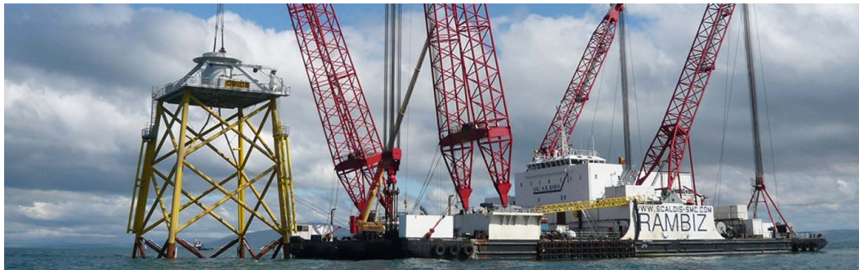
Figure 14. Rambiz 3000 lifting a transition piece in place (Deme-Group, u.d.)
