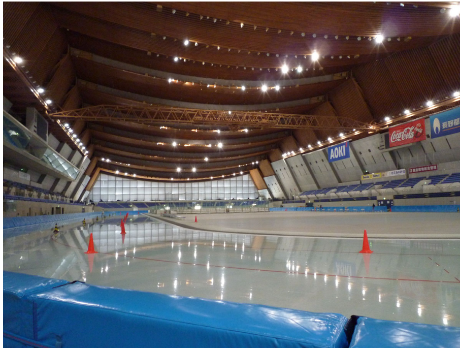
Figure 2.6: Nagano Olympic arena, showing the visitors experience of a catenary shaped roof Image source: Maclourin, (2017)
