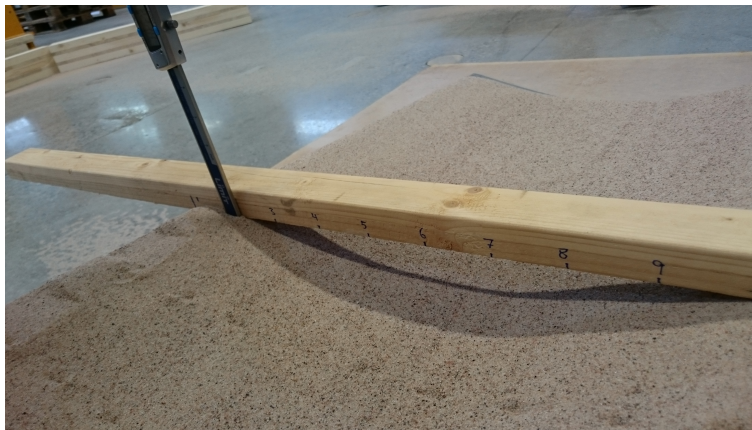
Figure 4.13: Method for taking point measurement over the roof
