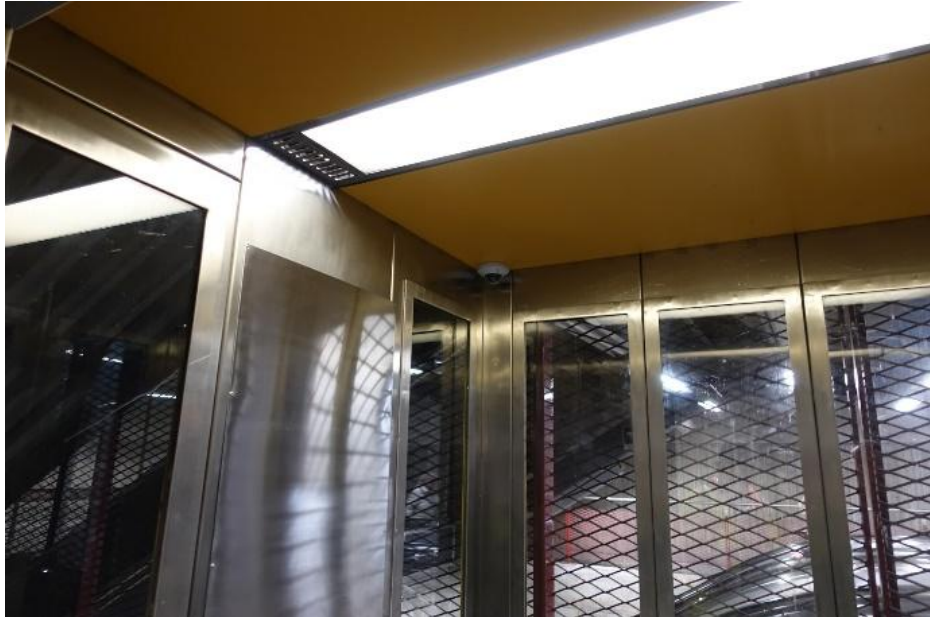
Figure G.2 The installed AXIS M3044-V camera in the elevator. [G.1]
