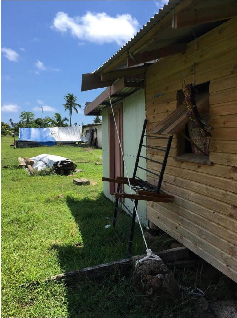
Figure 26: Rope and rock being used for keeping roof connected to house during hard winds
