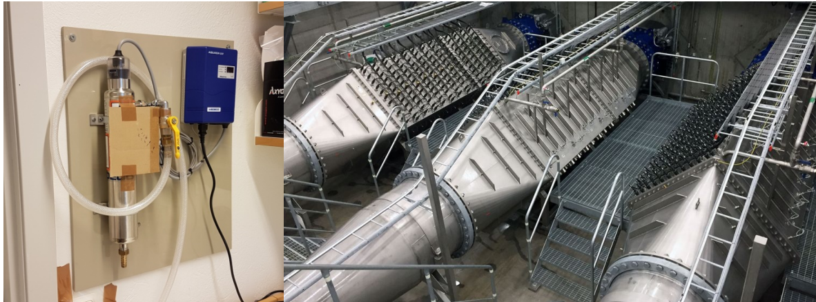
Figure 8. Labscale UV aggregate at TMB (left) and full scale UV aggregate of Ringsjöverket (right)
