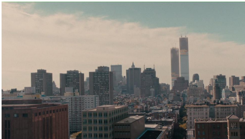
Figure 31 Wide shot of the NYC skyline, showing the Twin Towers in construction
