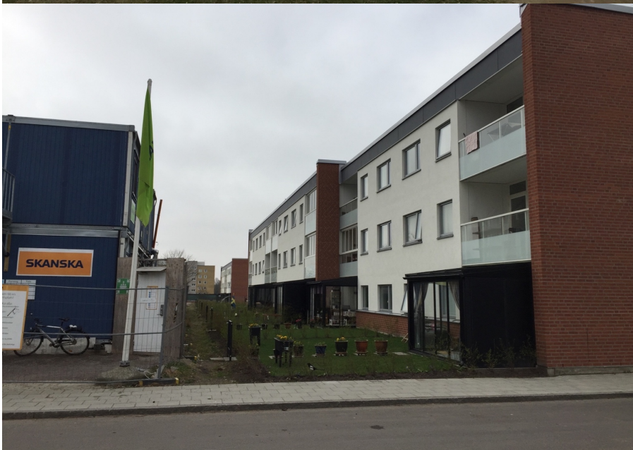
Figure 1. Illustrations of the renovation undertaken
