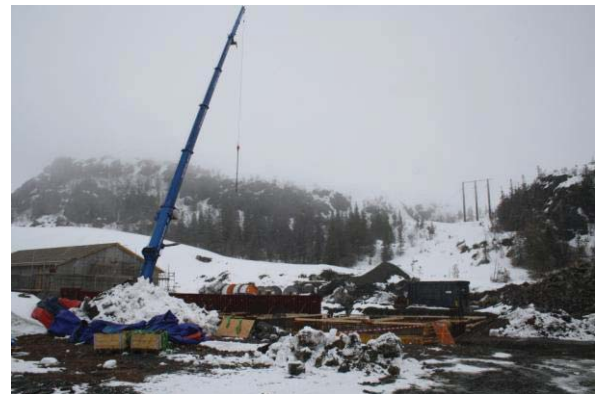
Figure 5. Construction of wind farm (own picture).
