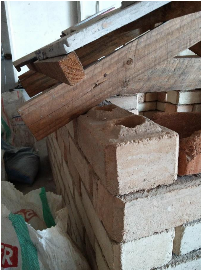
Figure 8 Soil-cement interlocking blocks stacked upon each other.
