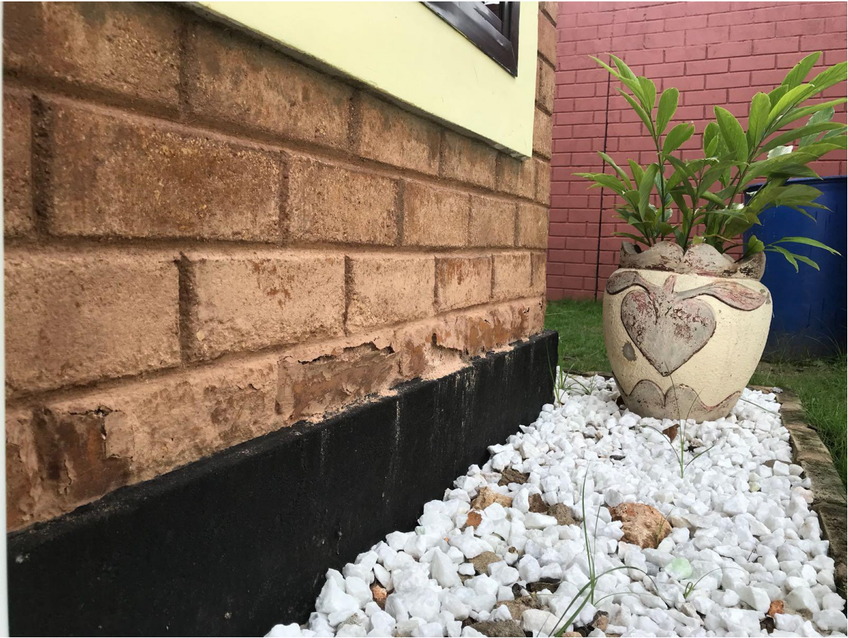
Figure 11 Moisture induced erosion problem
