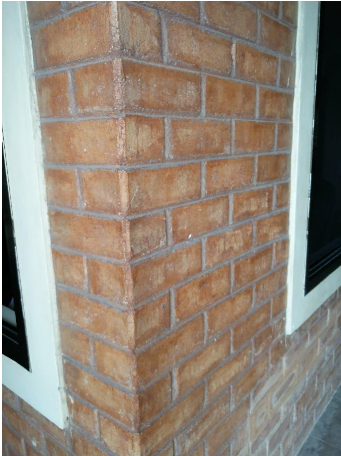
Figure 9 Finished wall with filled joints and polished face
