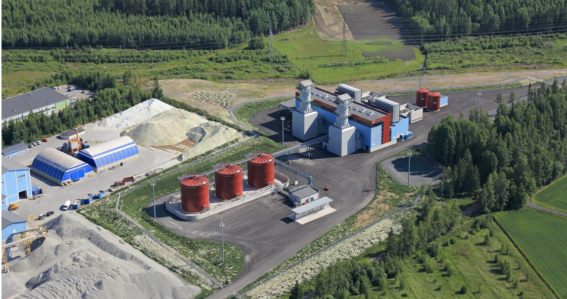
Figure 14: The 318 MW gas turbine facility in Forssa, Finland.
