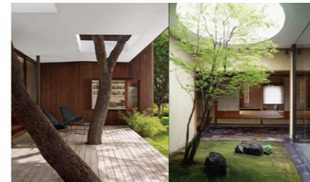
hole on the roof
