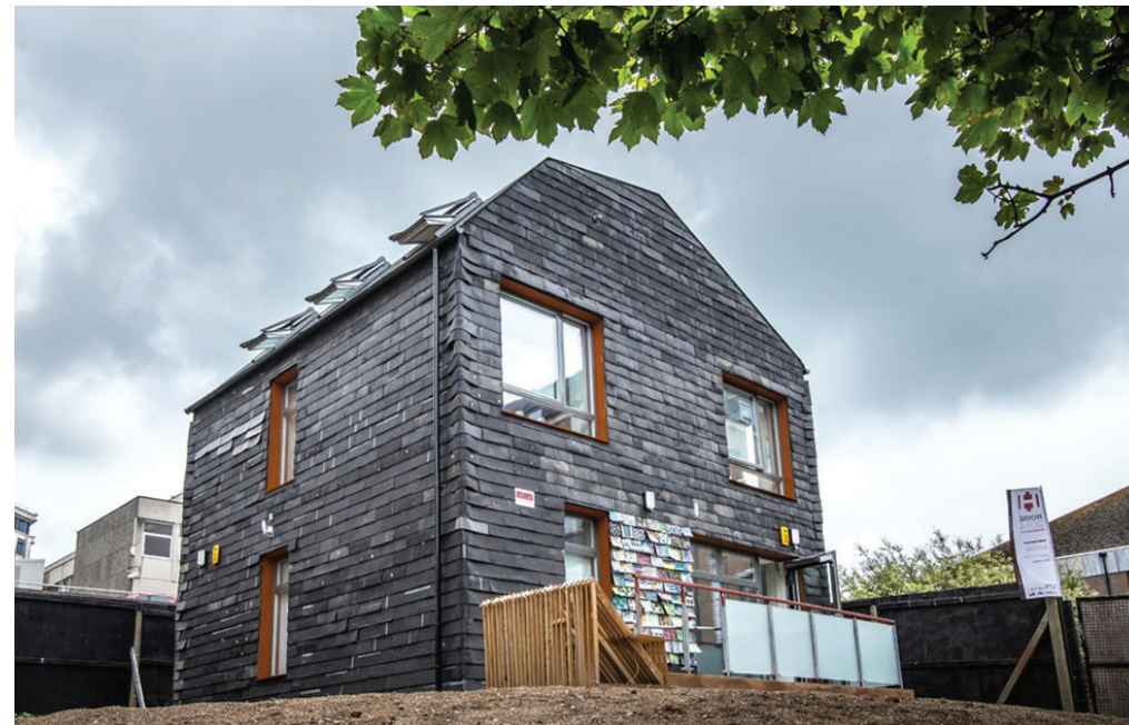
Brighton Waste House by BBM Sustainable Design
