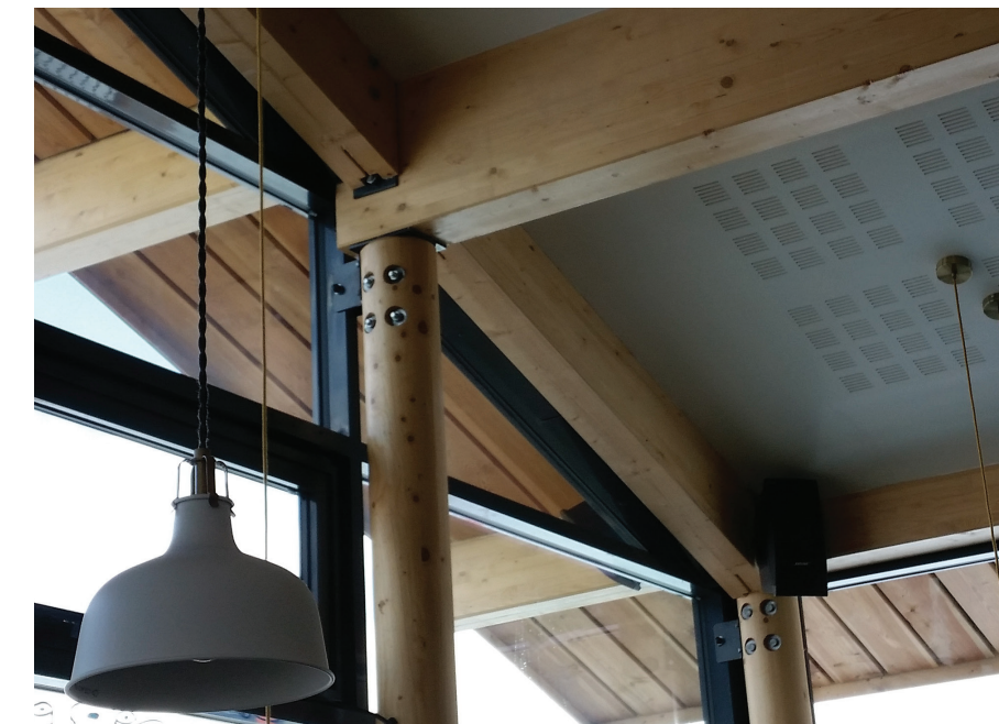
Example of non-permanent joint from a café in Les Arcs, France
