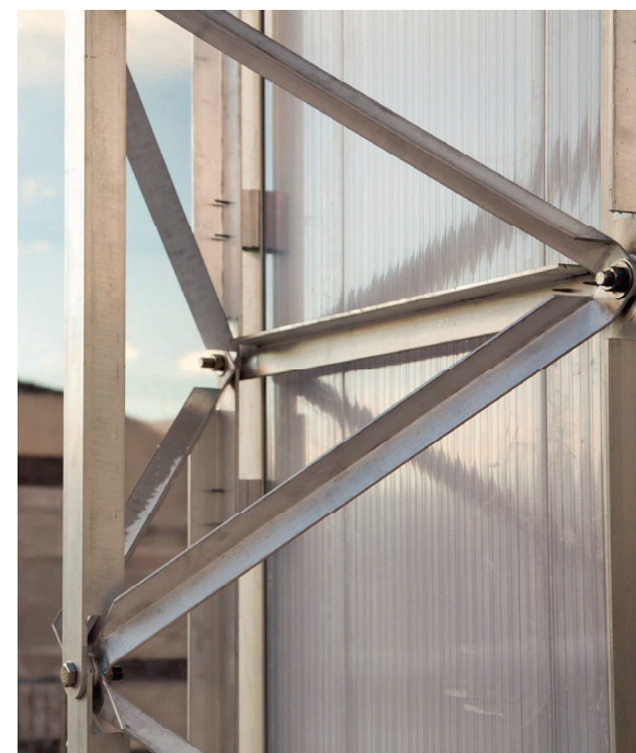
ICEhouse, close-up of the structure and its fasteners
