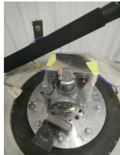
Figure 57: Fuel connector removed
