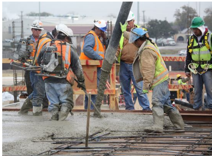
Tools of the modern builder, pouring concrete (Source: http://www.jbsa.mil/News/News/Article/462329/concrete-pour-underway-for-parking-garage/ )
