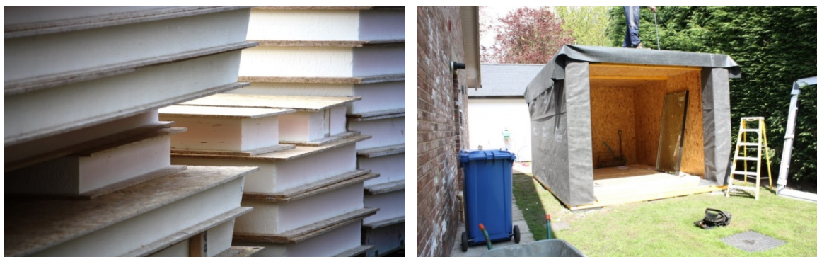
Figure 19. The SIP elements of SWIFT and a construction in progress (Source: http://www.swiftorg.co.uk/design-build/swift-materials/ )
