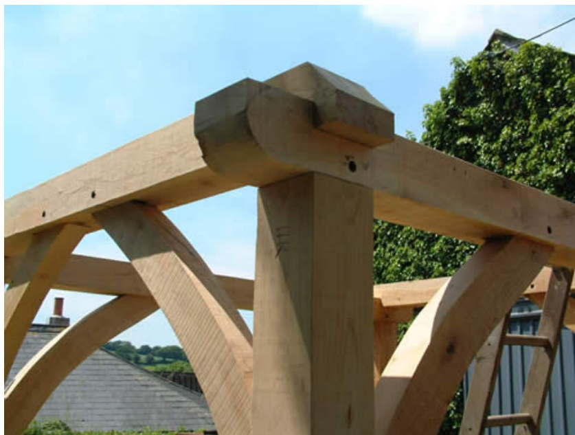
Figure 29. A traditional timber frame joinery construction (Source: http://blackcanyonbuilders.net/2011/12/07/timber-frame-joinery-a-primer-on-the-joints-of-timber-frame-construction/ )
