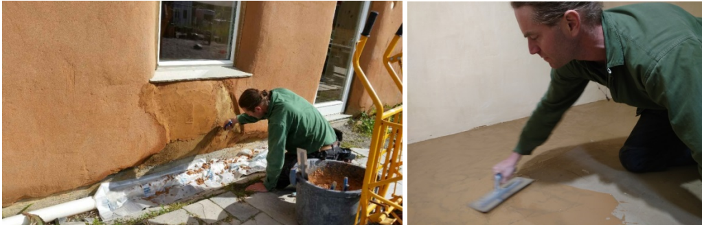
Figure 42. Wall reparation and floor laying using clay. Note the lack of protective clothing. (Photo: Julio Perez)
