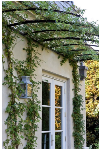
Figure 55. Trellis based shading method. Note that while in summer when the heating effect of the sun is highest the canopy of the plants protect the interior from overheating while in winter when leaves have fallen sun can freely penetrate through glazed surfaces and warm up the interior heat batteries (floor/wall surfaces). (Source: http://williamhefner.com )
