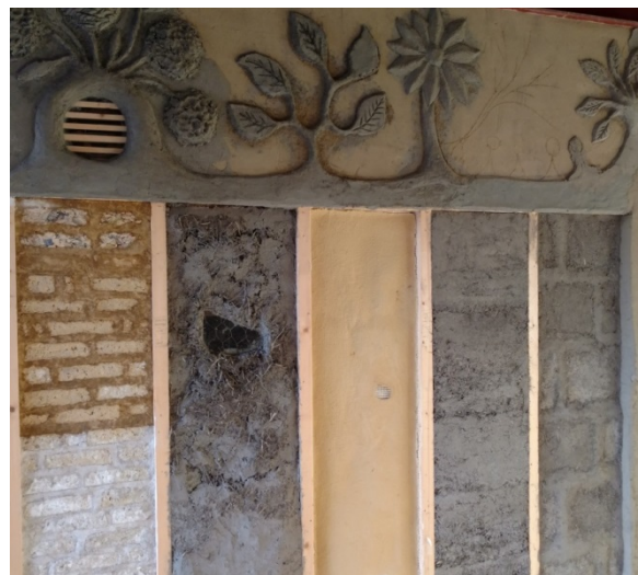
Figure 51. Clay walling techniques. The Clay Library at Gaia Architects, Nesodden, Norway. (Photo: author)
