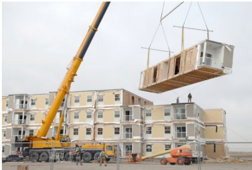
Figure 11. Placement of modules by crane in a construction. (Source: https://triumphmodular.com/blog/permanent-modular-construction/ )
