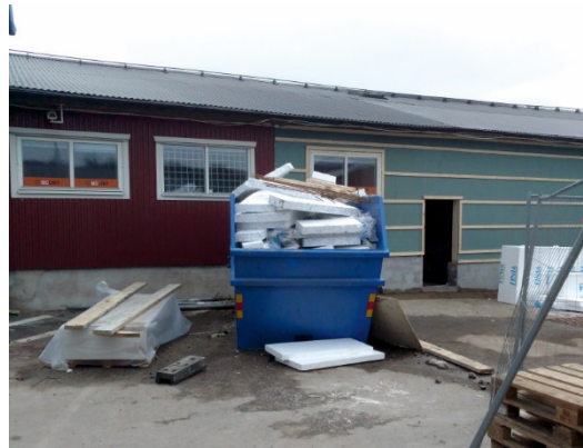
Figure 5. Waste at a conventional building site, March 2018, Norra Björstorp, Skåne, Sweden (Photo: Author)
