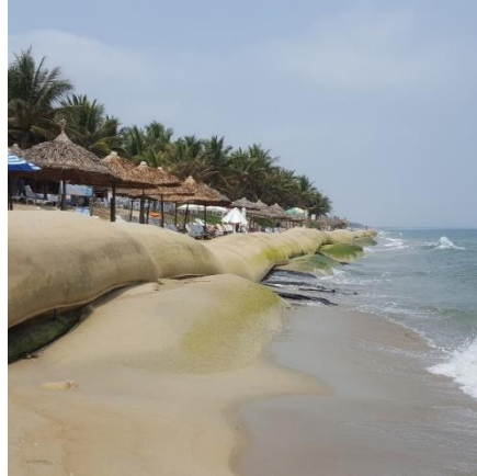
Figure 17. Protection with geotubes.
