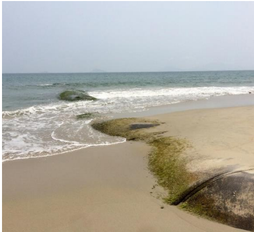
Figure 18. Groin made of geotubes.
