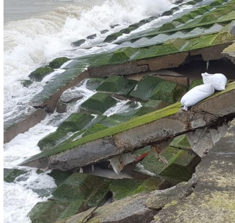
Figure 15. Damaged concrete structure.
