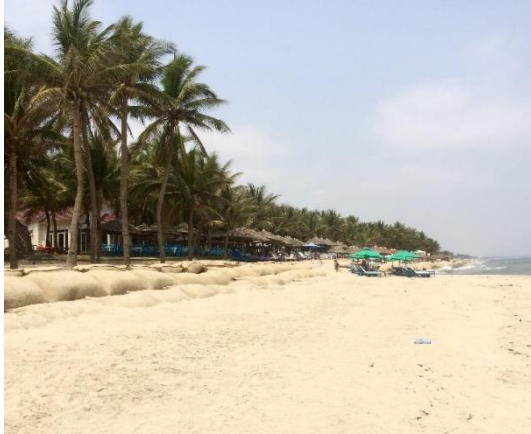
Figure 16. Protection with small sandbags.
