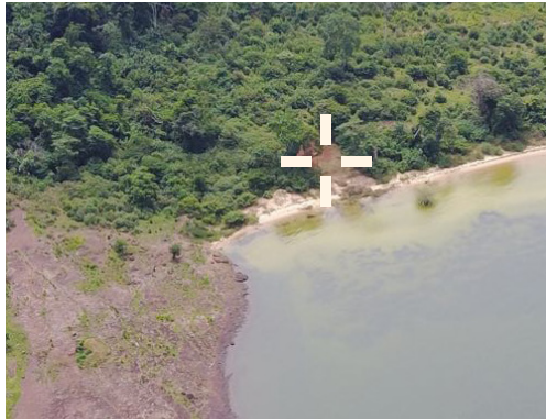
25. Aerial view of the construction site on Nsadzi island.
