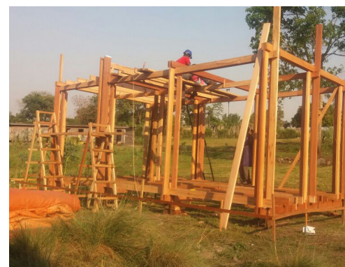
11. Roof ridge beam. The solution with a ridge beam was later removed as the system evolved.
