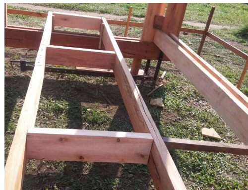
10. Blockings added to stabilize the joists
