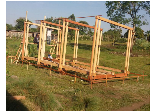
8. First ceiling beams
