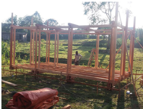
9. Secondary ceiling beams and floor joists
