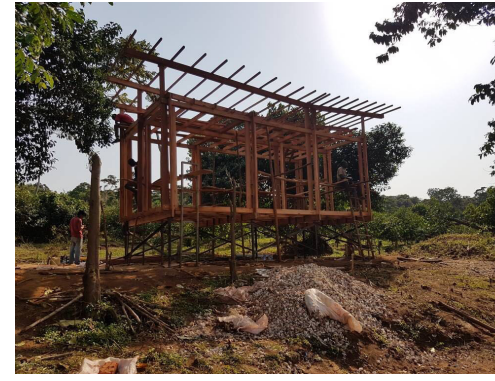
27. Most of the structure is reerected
