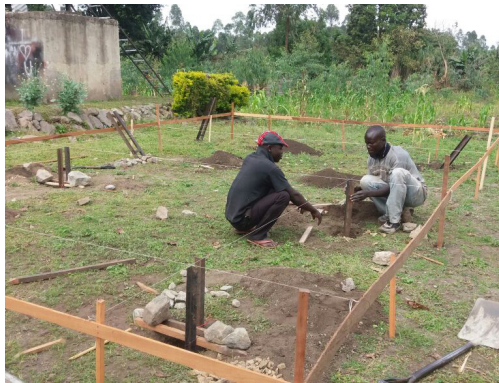
5. Setting out construction grid and footings
