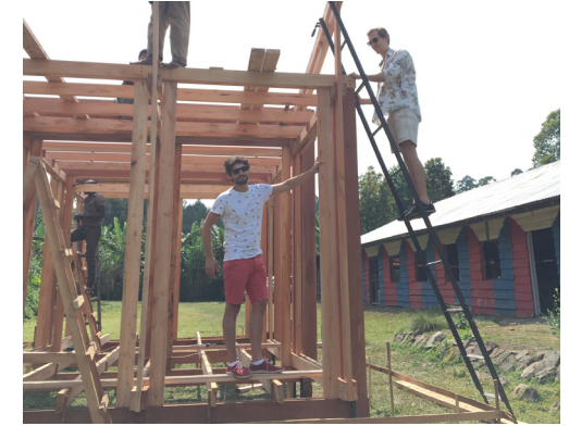
16. Clients and architect inspecting the proceeding work.
