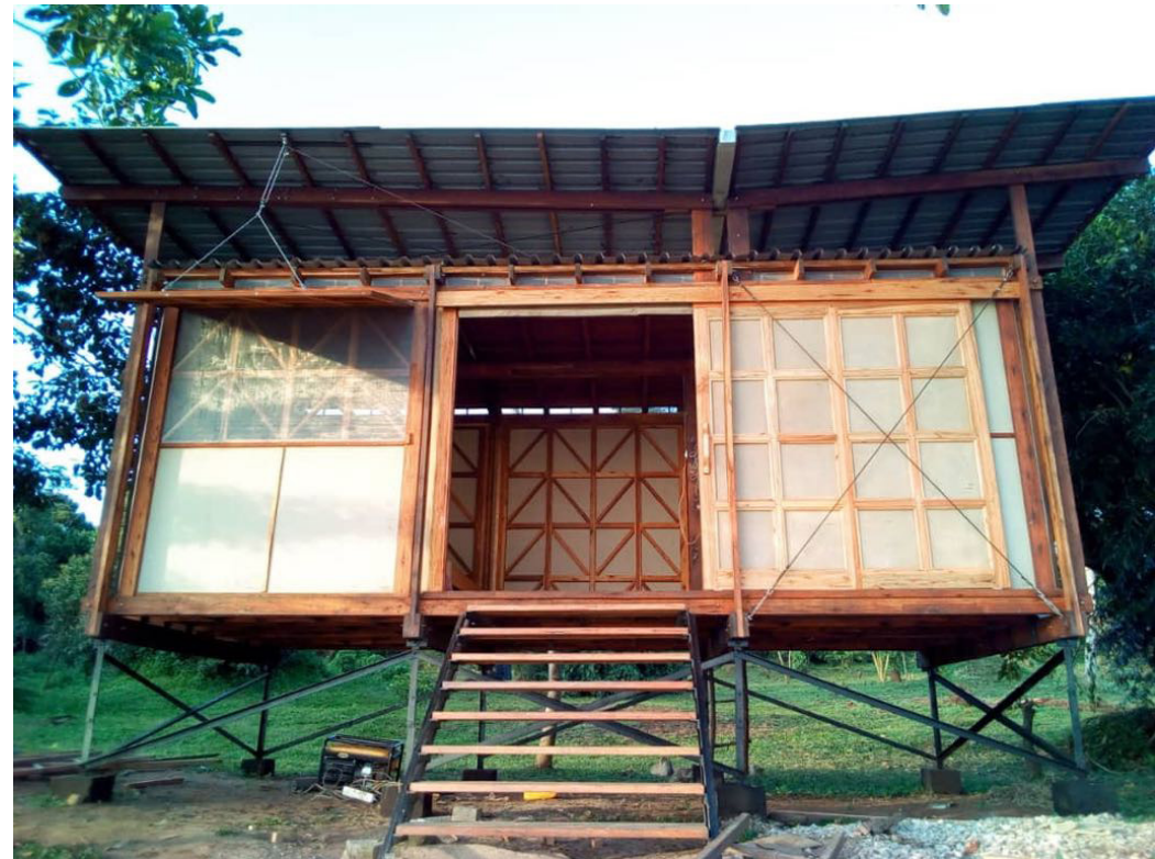
40. The sliding door are reinforced for more reliable operation.
