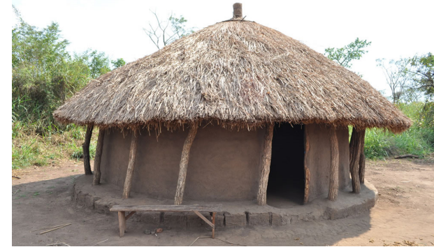
Wattle-and-daub hut with grass-thatched roof
