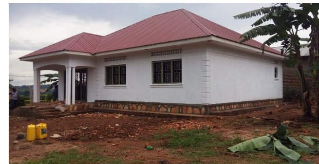
Brick or concrete masonry building with sheet iron roof
