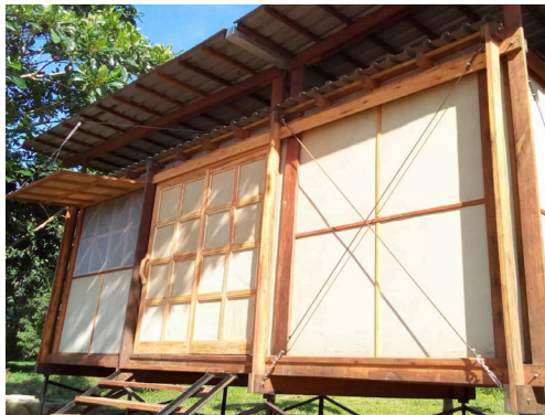
41. The bungalow's exterior is completed.
