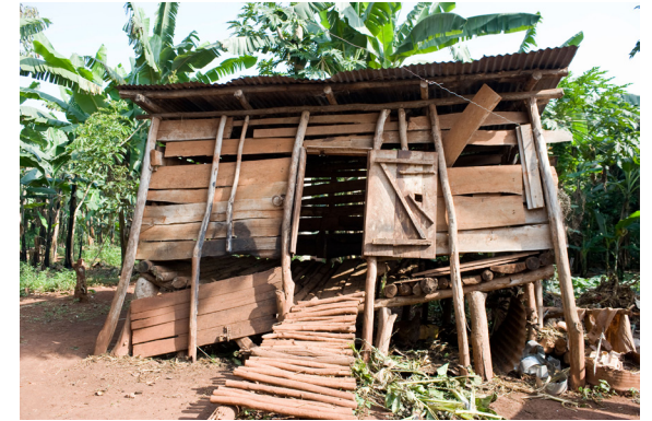
Rural shed with sheet iron roof
