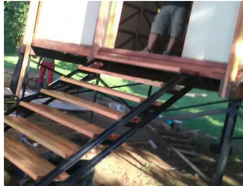
38. A way to access the bungalow: A stair.
