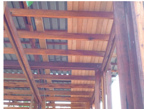
31. Ceiling and sub roof
