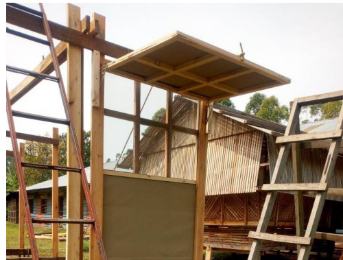
22. Window opening mechanism is being tested
