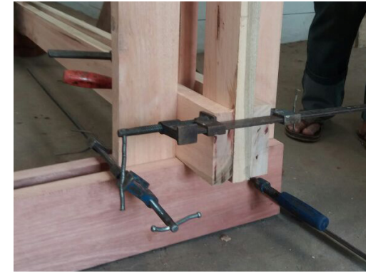
4. First mock up of the corner joint
