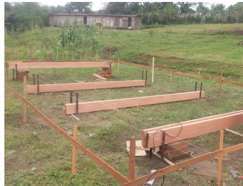
6. First floor beams
