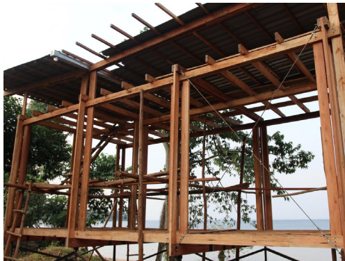
29. Roof, cross bracings and gutter almost in place.
