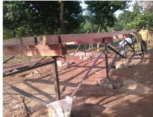
26. Concrete and steel footings
