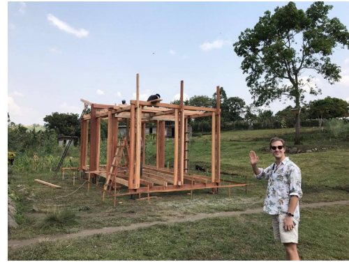
14. Seeing the structure for the first time
