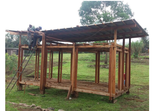
20. Corrugated sheet iron roof
