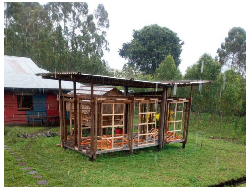
21. Wall panels are being tested
