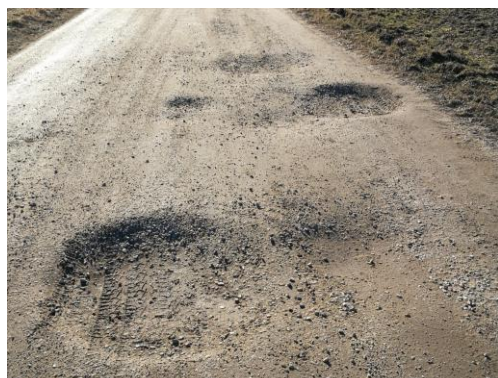
Figure 9 - An example of potholes in gravel road
