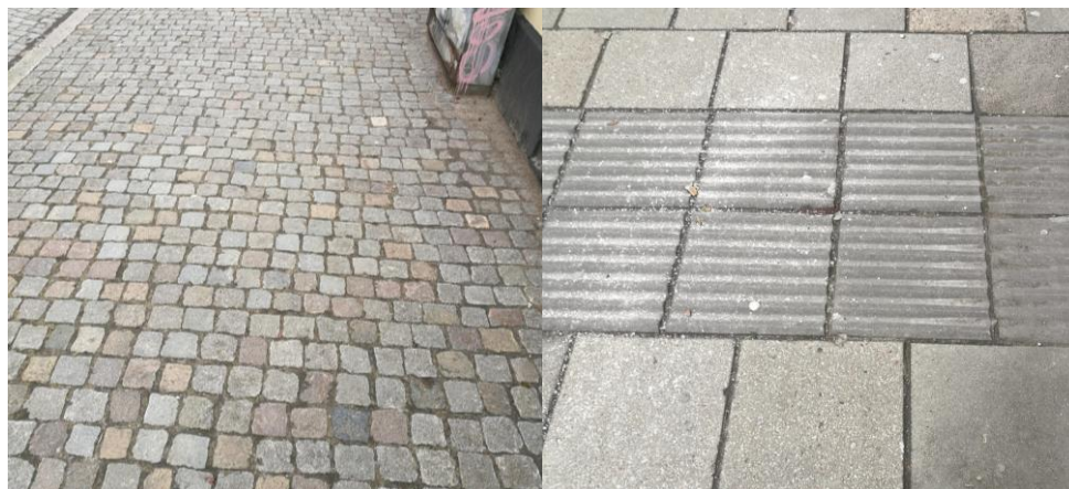
Figure 6 - Paving stone on the left, stone tiles with orientation pattern on the right
