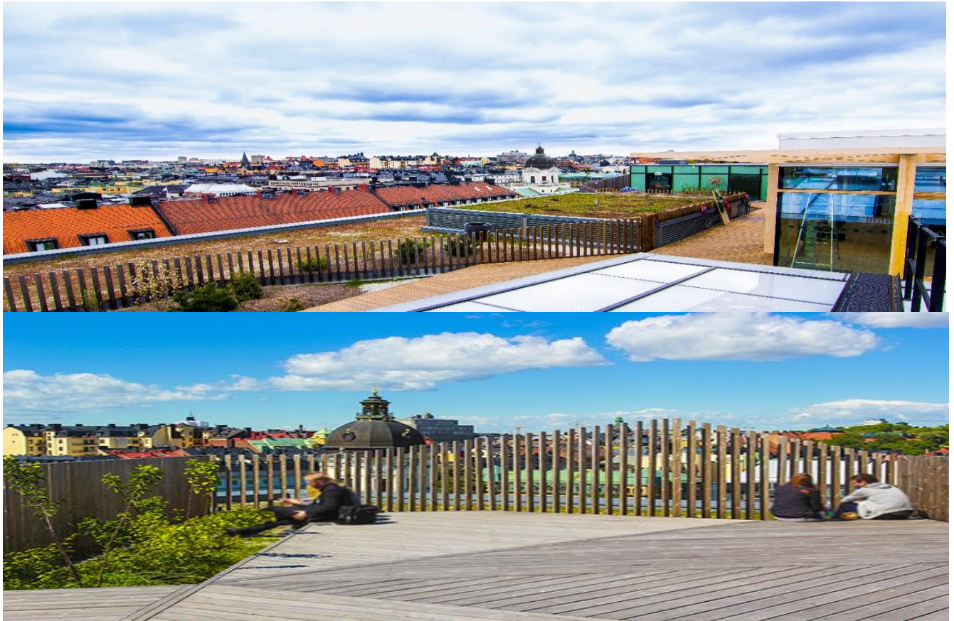
Figure 13. At Urban Deli in Stockholm, a green roof has been built which offers both social spaces and the ability to see far. A security fence with a 'natural' look keeps the visitors on safe distance from the edge of the building while also allowing vegetation to grow on both sides of the fence (Mynewsdesk, 2017).
