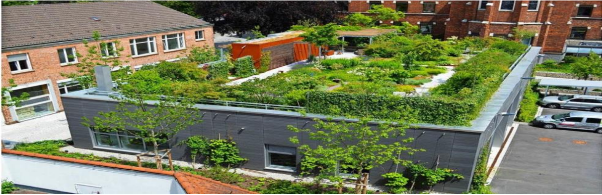
Figure 14. The roof garden of the Diakonissen-Klinik in Augsburg which both visually enhances the yard and improves stormwater management and the climate (Optigrün, 2013).
