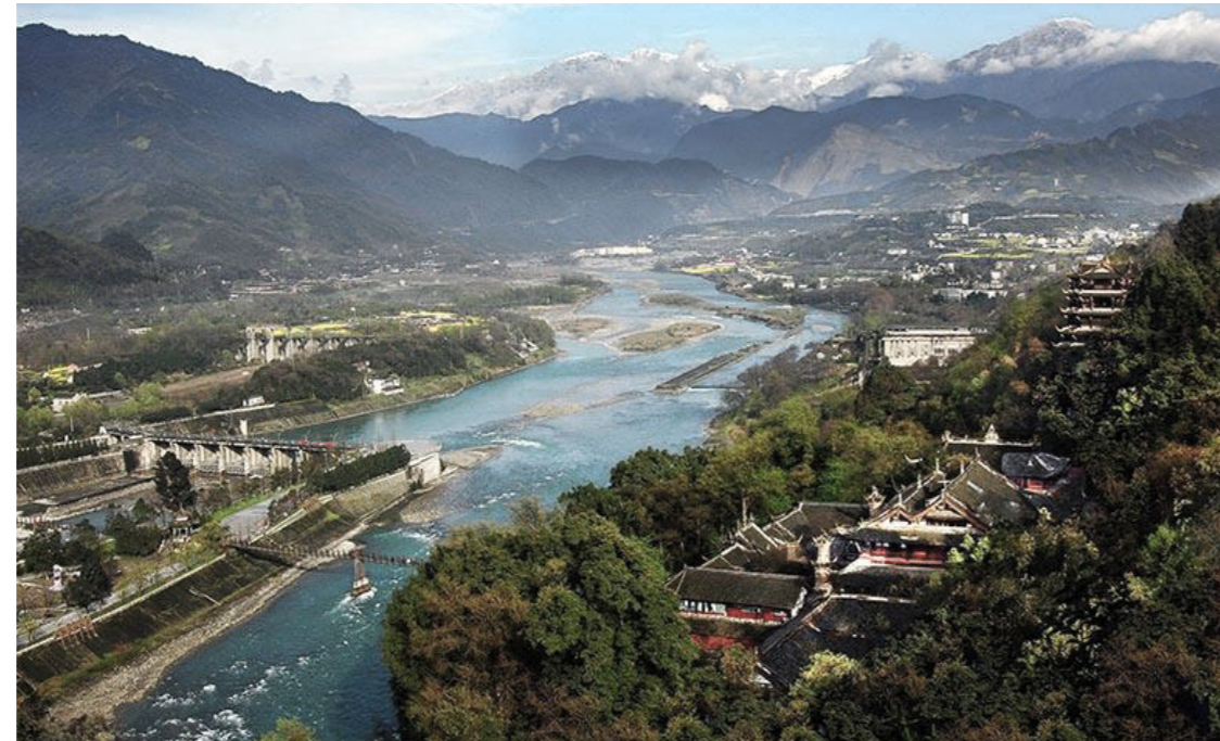
Irrigation System, Dujiangyan
