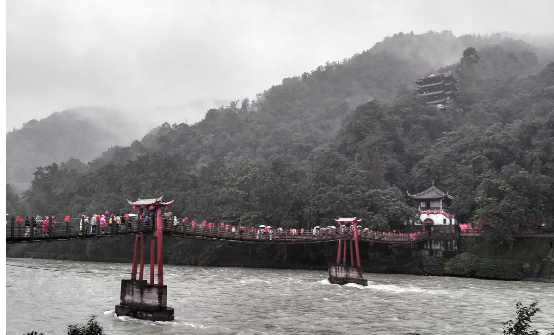
Anlan Suspension Bridge, Dujiangyan
