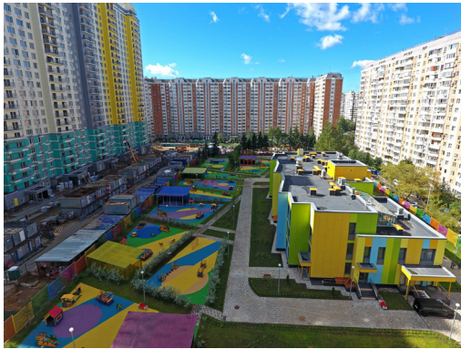
Fig. 23 Newly opened kindergarten, Moscow
