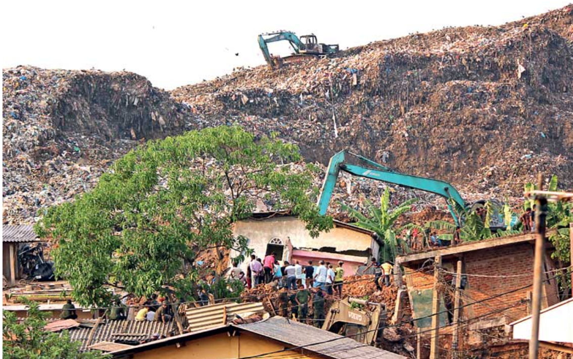
Figure 2-5 Garbage mountain collapse
