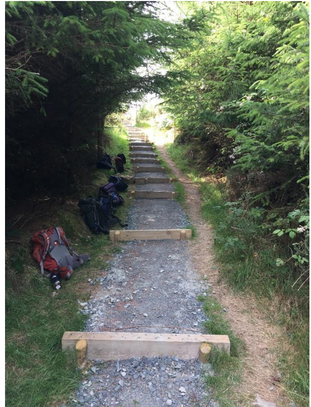
Figure M-2 Steps built by MM 2017 on path between Wicklow Way and Avonmore Way
