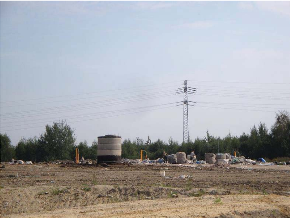
Figure 6. Landfill gas collection and waste picking activities. Behind is the future location of the biogas plant (SPSEP).
