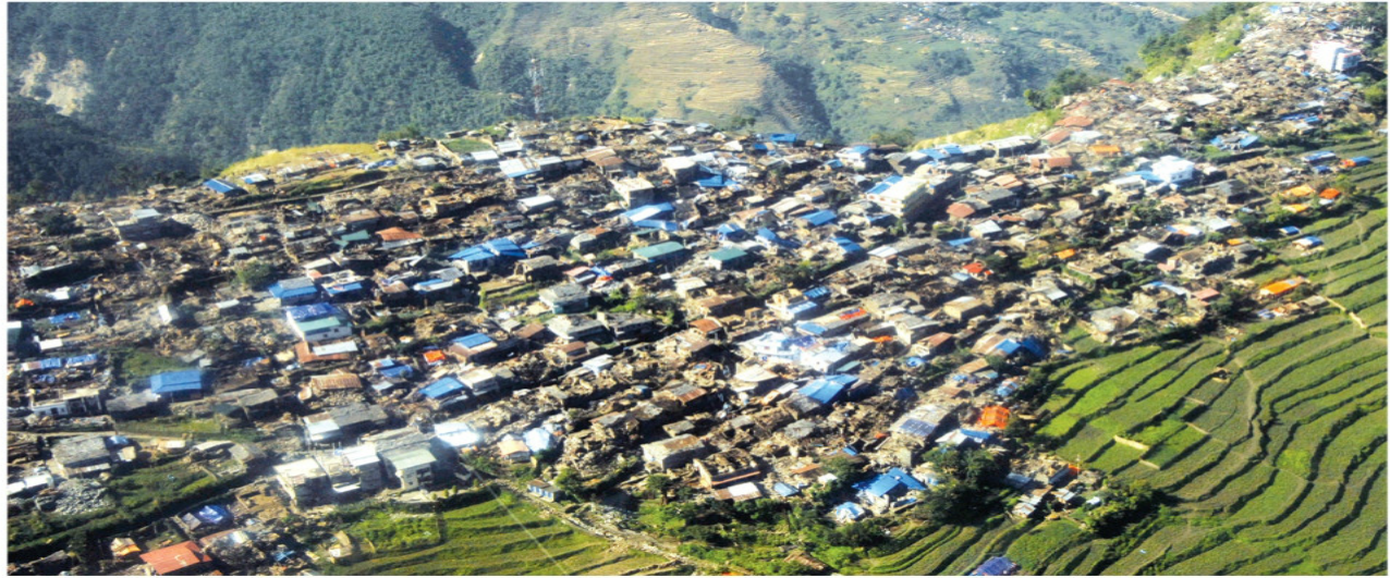
An aerial view of Barkpak village in Gorkha district, the epicentre of the devastating April 25 earthquake.
