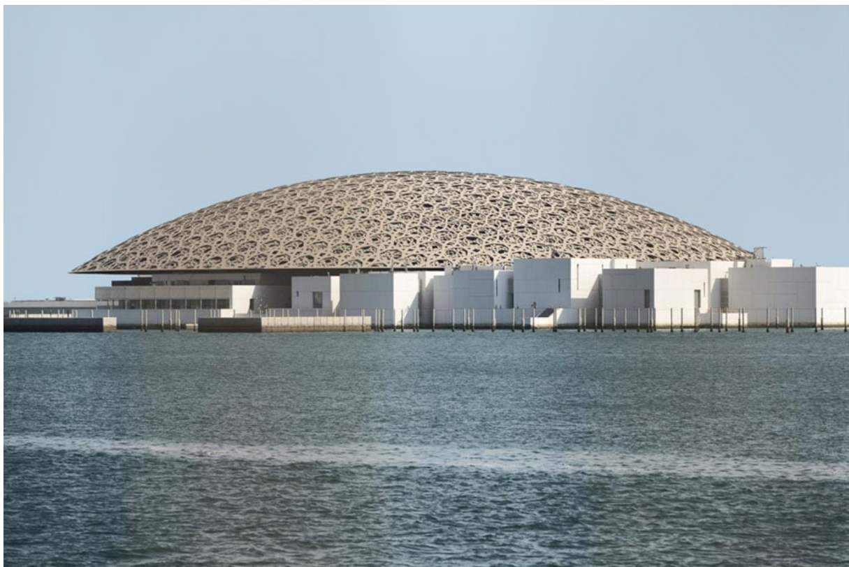
Foto 5. Jean Nouvel, Louvren Abu Dhabi, 2017, Abu Dhabi.
