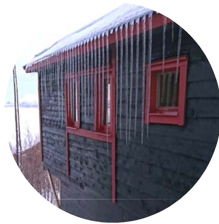
Icicles Forming on the Cabins due to Inefficient Insulation
