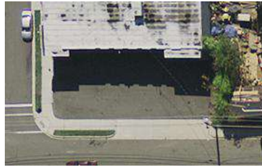
Figure 3.1: An example of a parking lot without any visible parking spaces.
