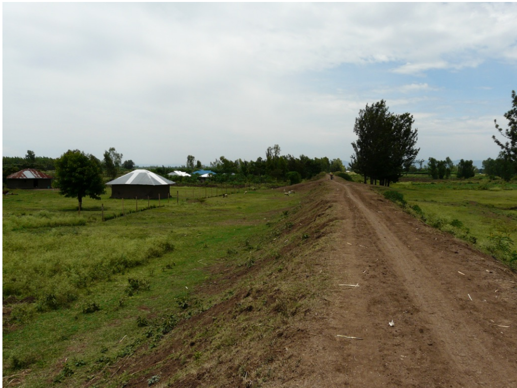
Figure 12. Built walls along River Nyando.
