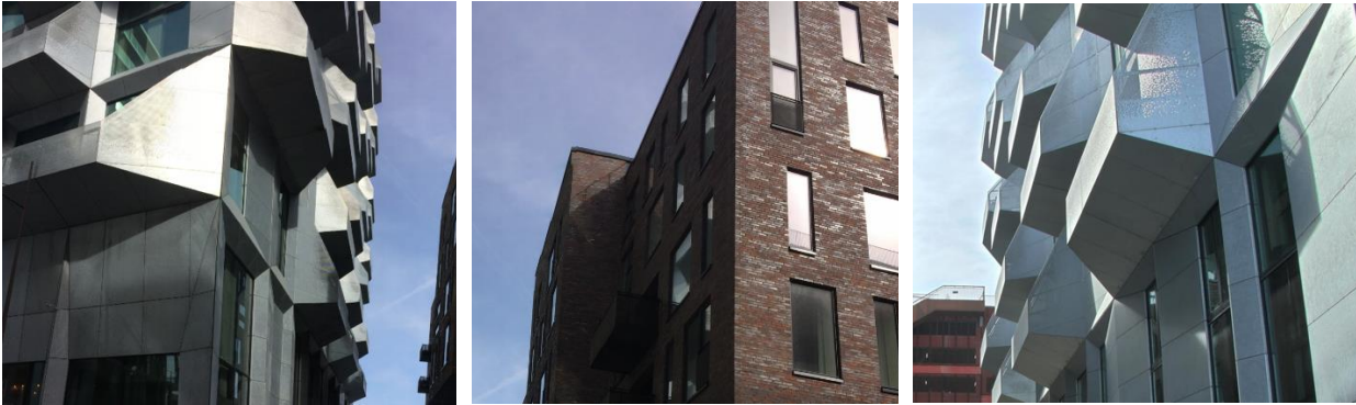
Figure 23 Images of glare – canyon A: left – metallic façade, center – glazed window; right – transparent metal grid.
