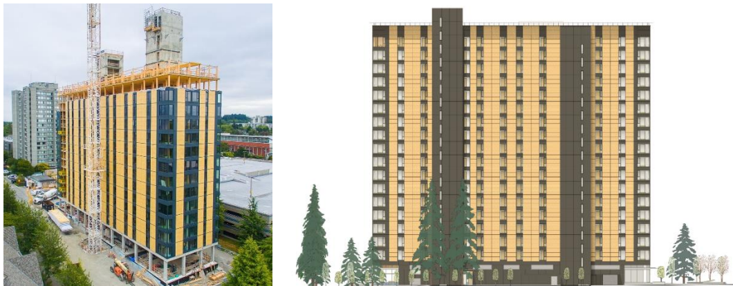
Figure 13.4: Brock Commons Student Residence (Canadian Consulting Engineer 2016; Acton Ostry Architects and the University of British Columbia 2016).
