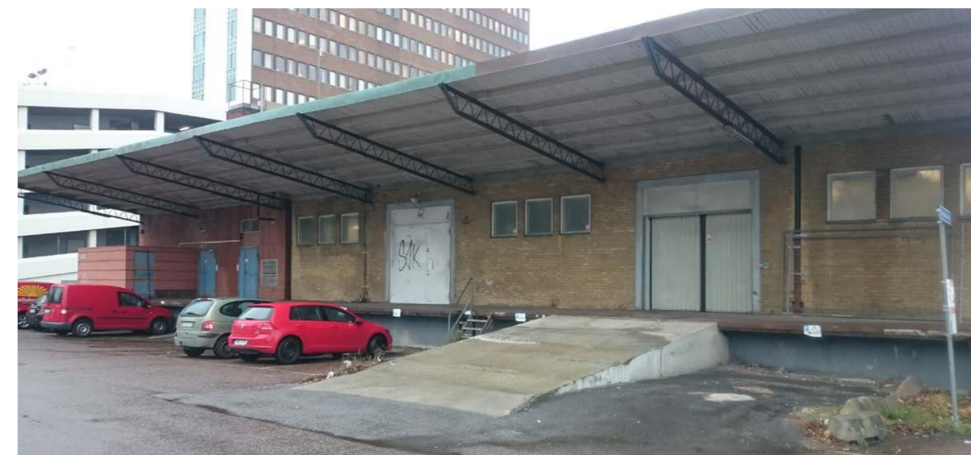
Figure 42. Storage building, Nyhamn malmö ,Taken by:Hany elhassany
