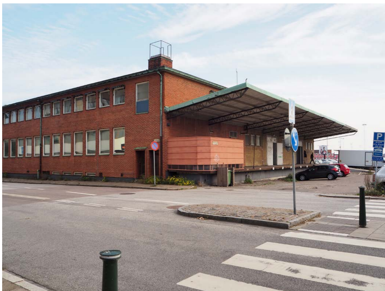
Figure 138. Image of the storage building
