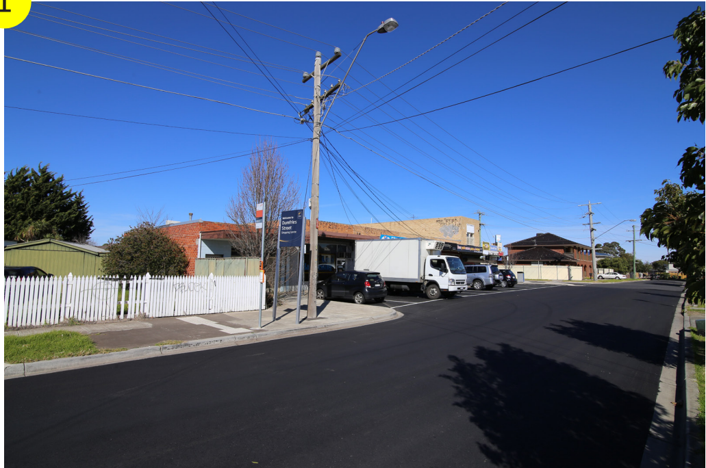
Right: View to shops from the north with bus stop in foreground
