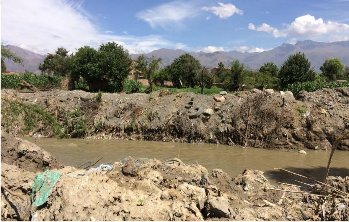
Figure E. The Rocha River at ID 6, showing banks that prevent flooding and solid waste deteriorating
