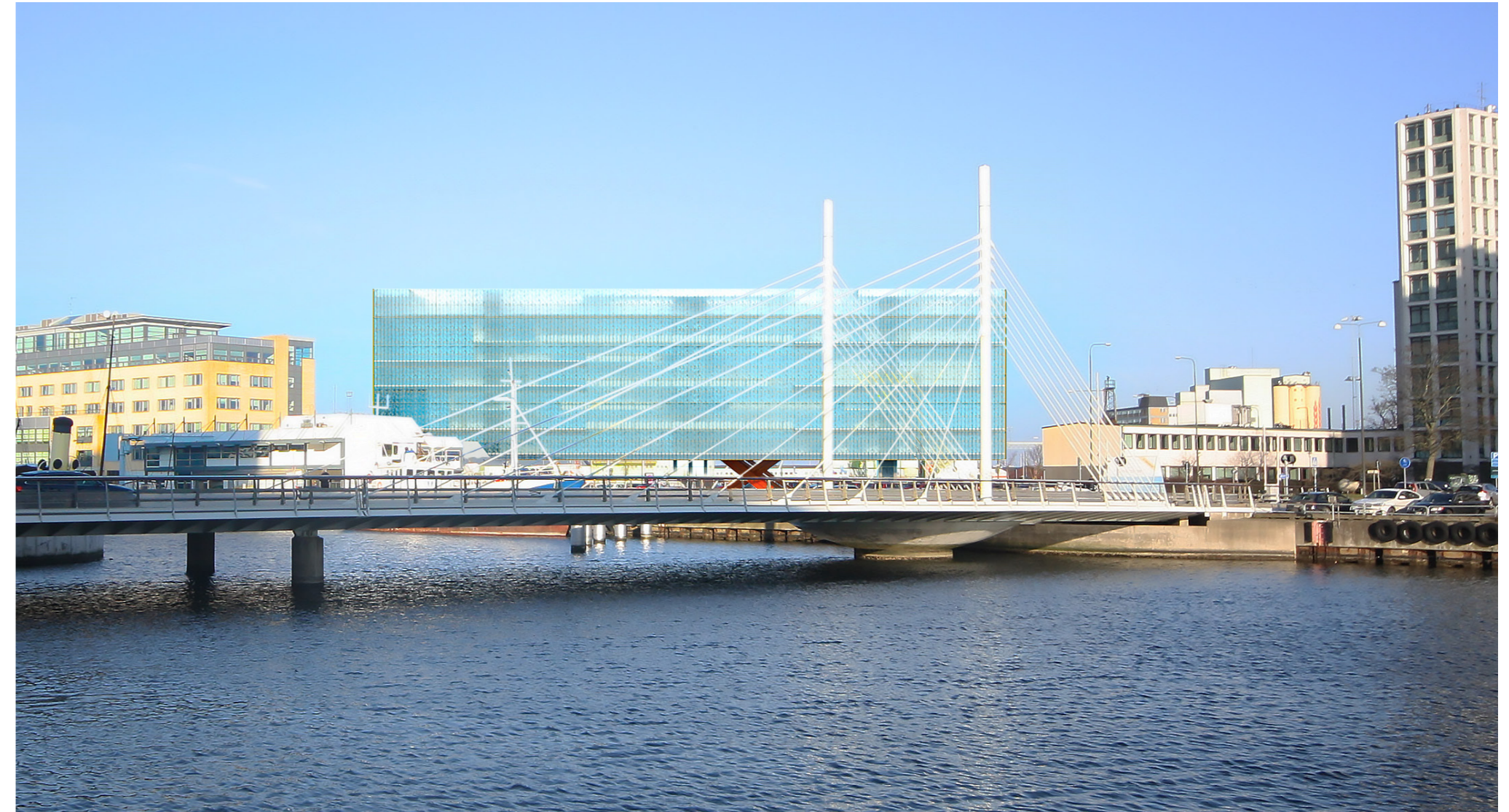
The Pier seen from Malmö University
