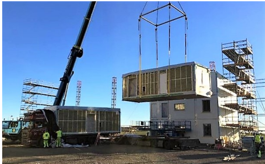
Figure 2.1: Module lifted into place at a TVE building site.
