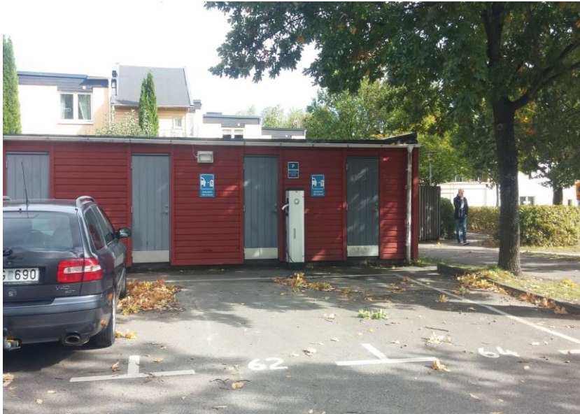
Figur 27 Laddstation Spexaren ga:1.
