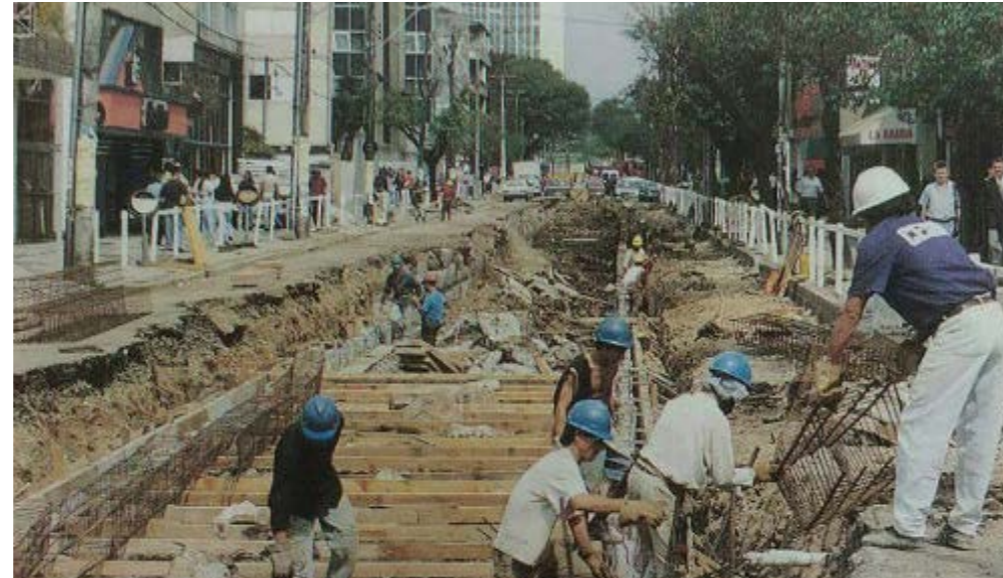
Channeling and covering of the rivers
