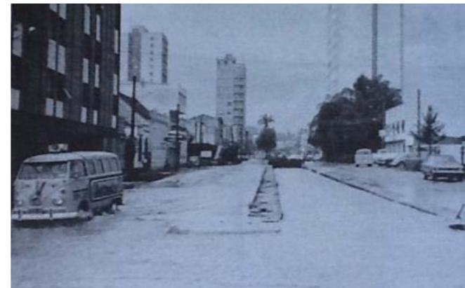
Mariano Torres street flooded before the covering of the Belém river
