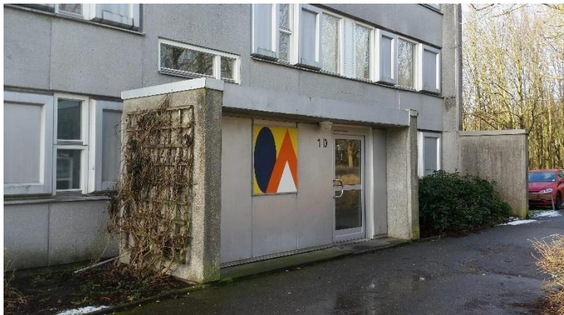
Figure 2: One of the entrances facing north (photo taken by the authors).
