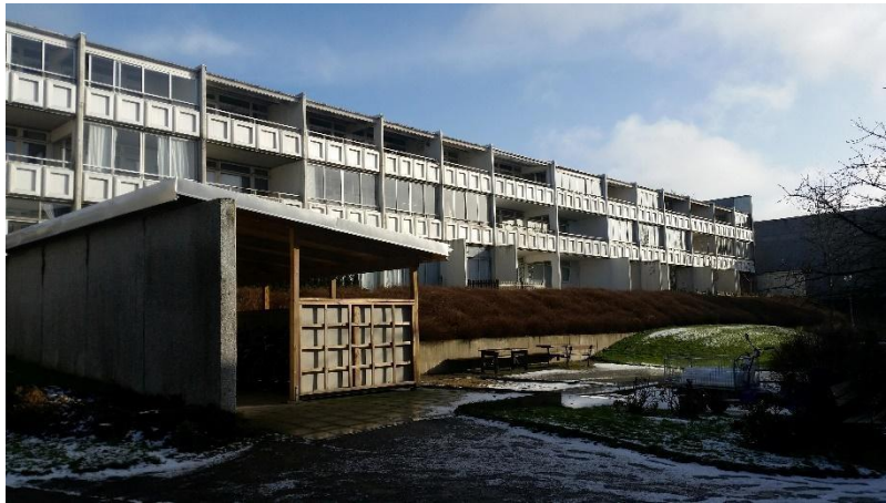
Figure 3: The south facing façade (photo taken by the authors).
