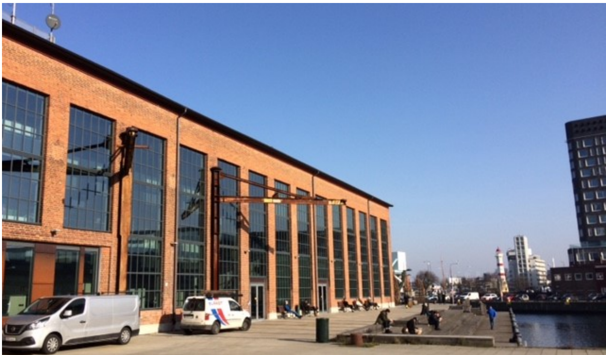
Figure 5: A wharf in Varvsstaden, behind the converted offices of 'Sveriges Television AB' (Author's own, 2019).
