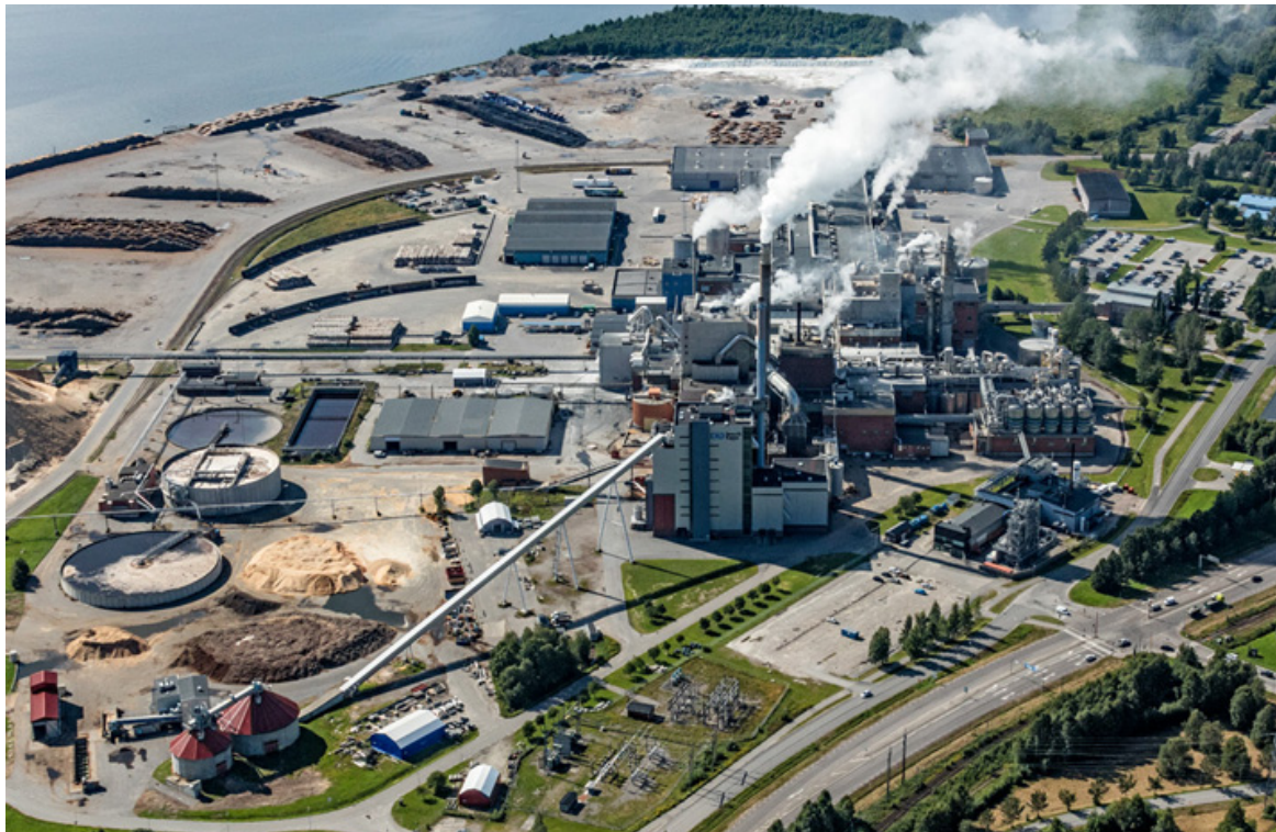
Figure 2.5. Aerial photograph of the Smurfit Kappa paper mill in Piteå, Sweden (Smurfitkappa.com, 2018)
